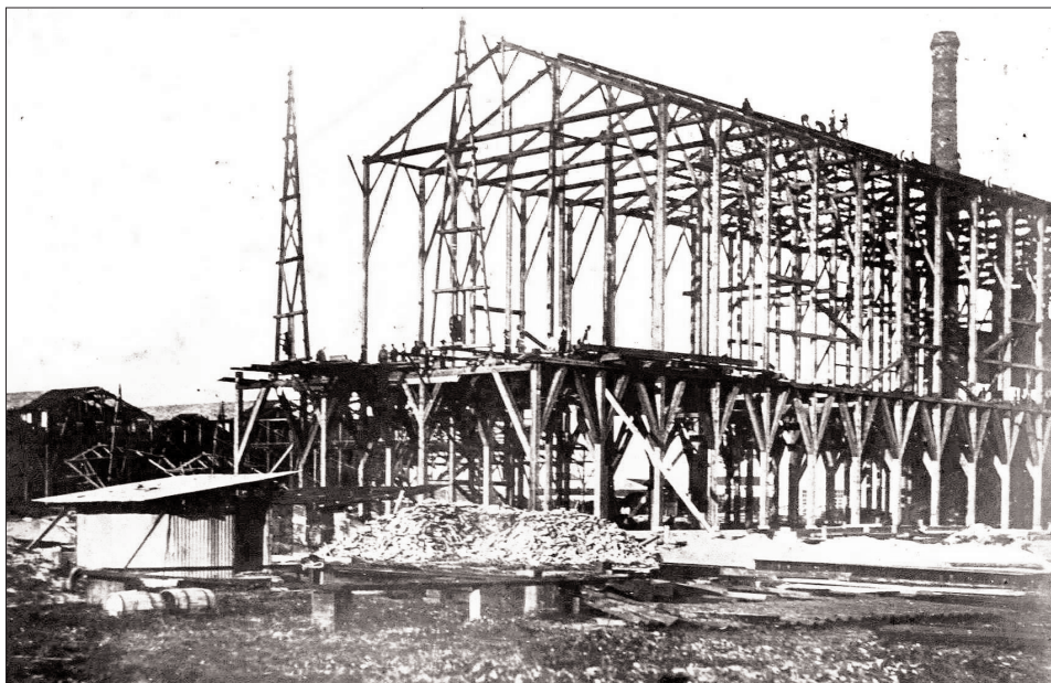
The plant at Barreiro under construction (1906-1908).
